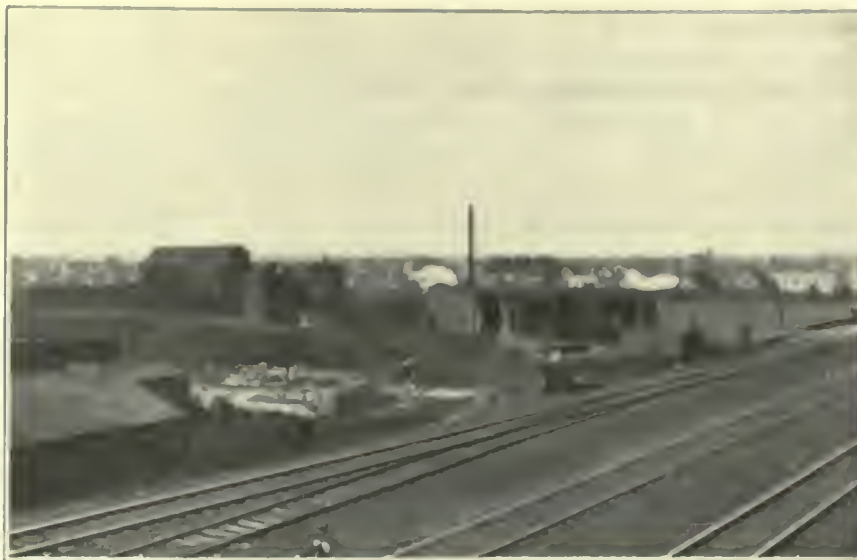
FIG. 350. LOCOMOTIVE TERMINALS. Engine House of the Chicago Great Western Railroad at 46th Avenue and the Baltimore & Ohio Chicago Terminal Railroad.
